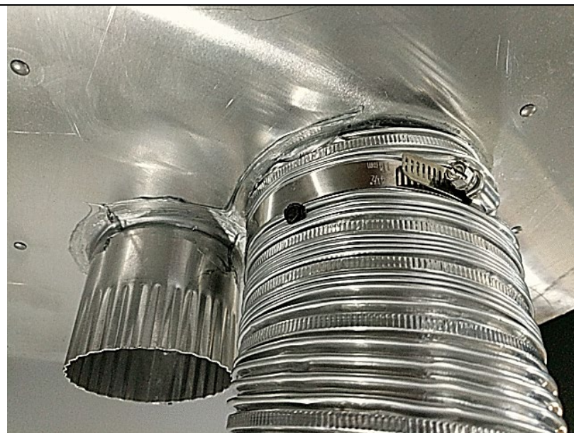
Vent Cap Flex Connection Hose Clamp first. Secure w/ Screw above Hose Clamp
